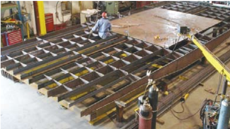
MAJOR FABRICATION ↗ Replacement ramp for car ferry.
